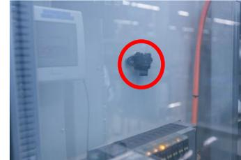
Measurement of humidity, temperature and smoke, air pressure, etc. for electric cabinet
